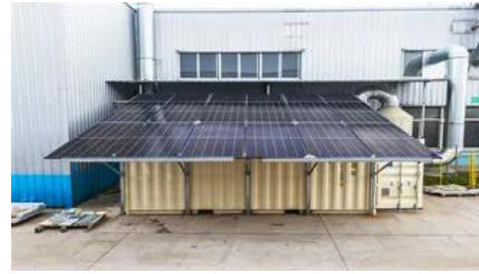
Fortress Power eSpire Nano Commercial Energy Storage System
