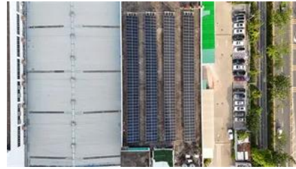
The Power of 10 lands at Datacenter World, Austin, Texas
