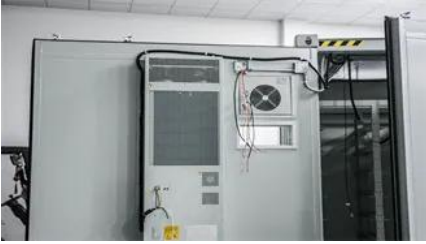
South Ossetia Mobile Energy Storage Container 20MWh
