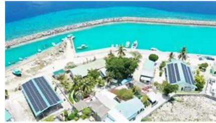
500kW 1MWh Microgrid Industrial Battery Energy Storage System
