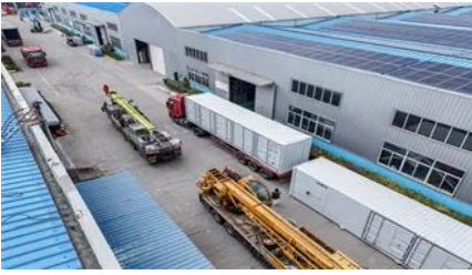
50kW/100kWh Battery Energy Storage System Pakistan
