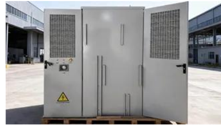
China's CGN Breaks Ground on Laos' First Big Solar Power Project
