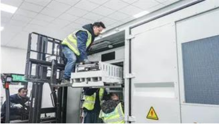
Custom Outdoor Electrical Cabinet , Inverter & Battery
