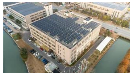
Energy storage container customization factory in the
