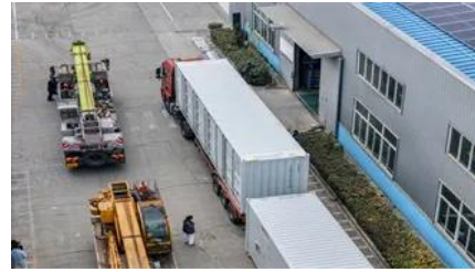
Utility-scale battery energy storage system (BESS)
