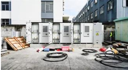
373kWh Liquid Cooled Energy Storage System
