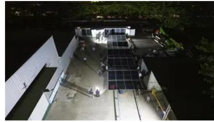
10KW solar power system installation in Hungary.
