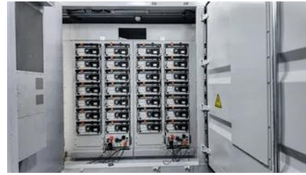
SolaX ESS-AELIO , C&I Energy Storage ESS Cabinet , 50kW/60kW
