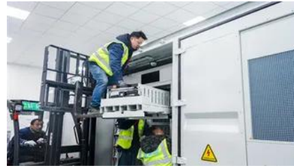
500kW Niger Mobile Energy Storage Container for Farms
