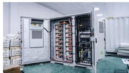
Alibaba : ZLPOWER IP65 Battery Cabinet, modular design and
