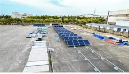
Envision Solar , Solar Panel Installation , Phoenix AZ
