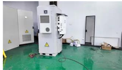
Li-Ion Battery Storage solar power system.
