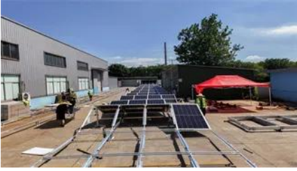
Envision Solar , Solar Panel Installation , Phoenix AZ
