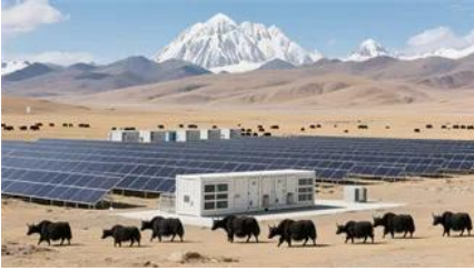
Phoenix Solar Company , Argent Solar Electric
