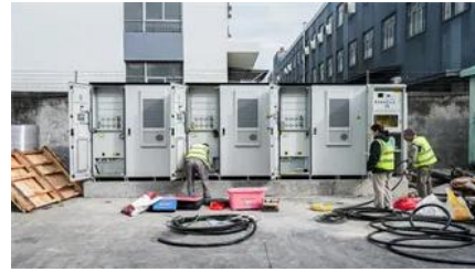
200 kWh Battery Energy Storage System , BESS Cabinets
