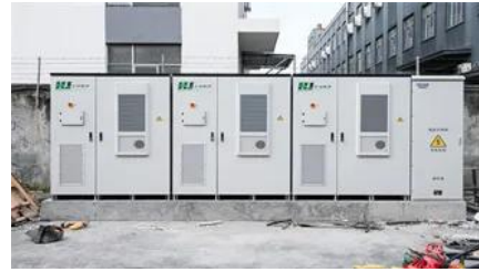
Vaduz outdoor energy storage power supply communication
