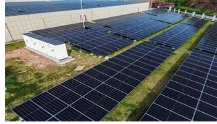
Communication site energy cabinet management system
